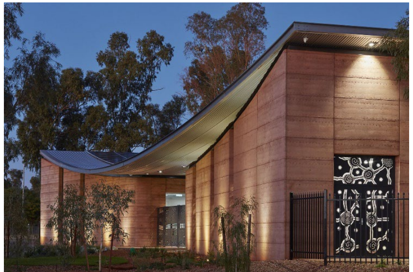
Newman Clinic and Administration Building
